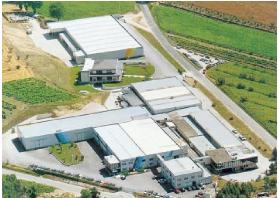
Massa Martana plant: air view
